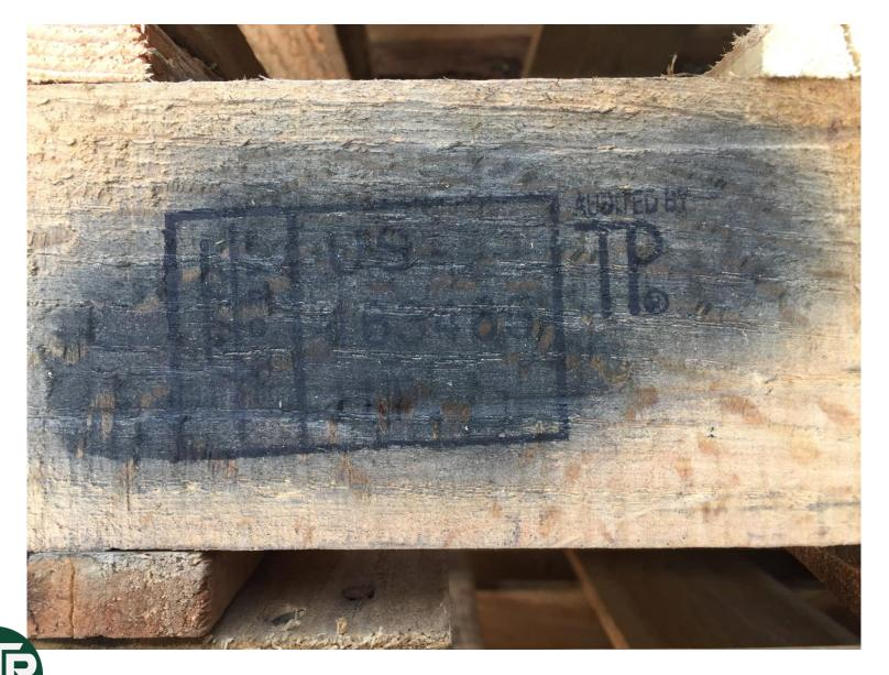
This mark is NOT obliterated since it can be seen through the paint...NON-CONFORMING!
